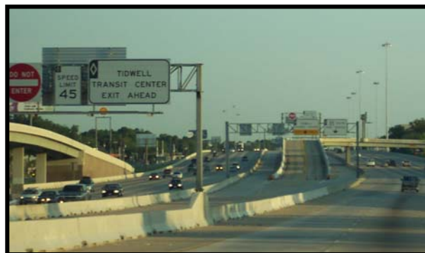
US 59 North HOV Facilities
